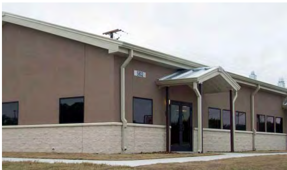
DoD IG recommended Army officials create working groups to implement GFEBS functionality necessary for Army real property management.
