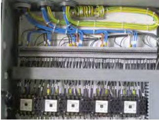
DoD IG identified electrical hazards during a site visit in Afghanistan.
