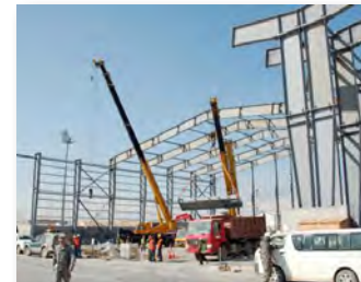
DoD IG reviewed military construction projects in Afghanistan.
