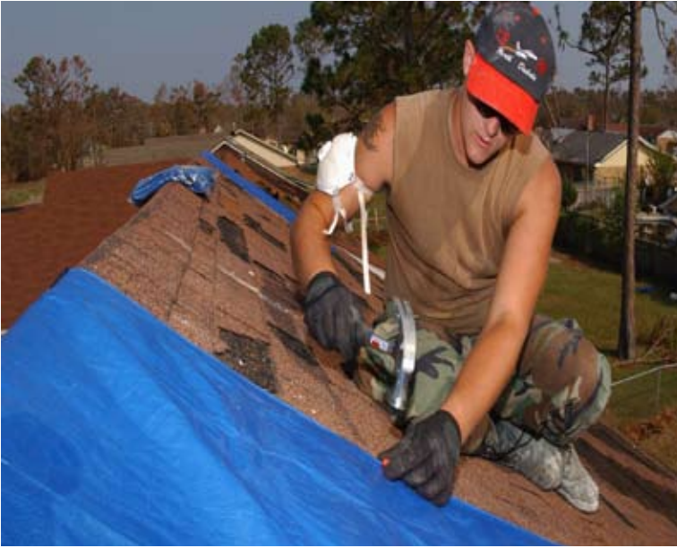
An Air Force senior airman nails a cover on a roof of a home damaged by Hurricane Katrina.
