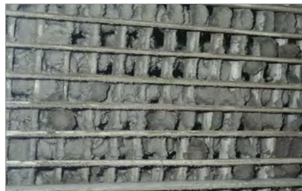
Military Housing—Clogged Air Return Registers DoD IG photo
